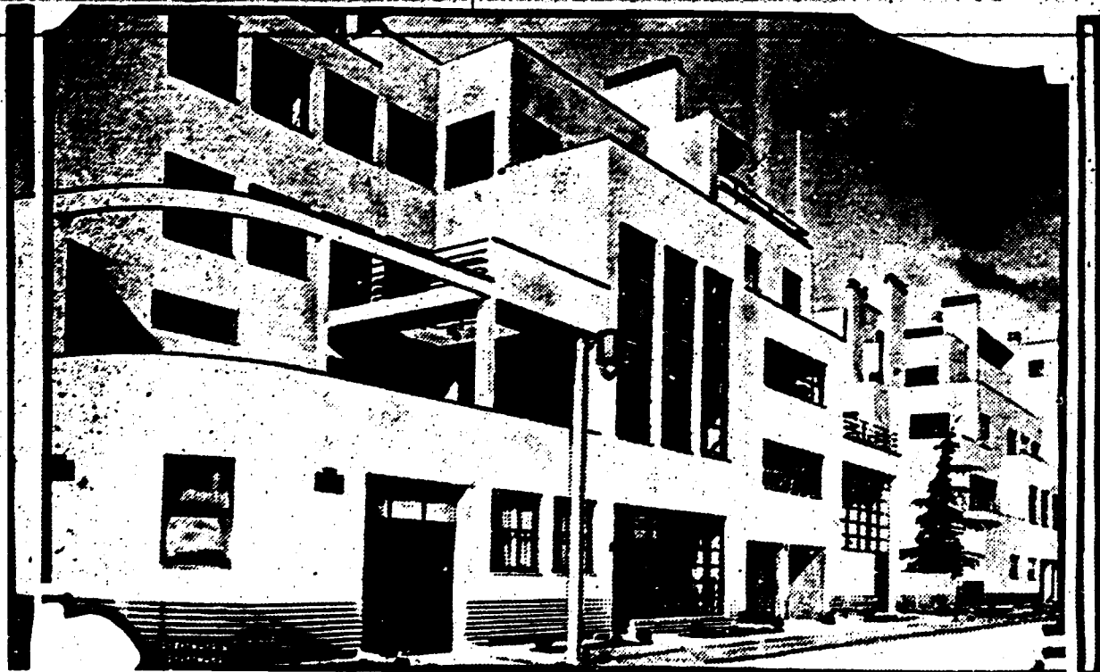
Decks of the big transatlantic liners are the inspiration of the first ultra-modern street of Paris, the Rue Mallet-Stevens, built by and named after the brilliant young French architect who heads a new school of designers of buildings. The entire street is built in white cement.
