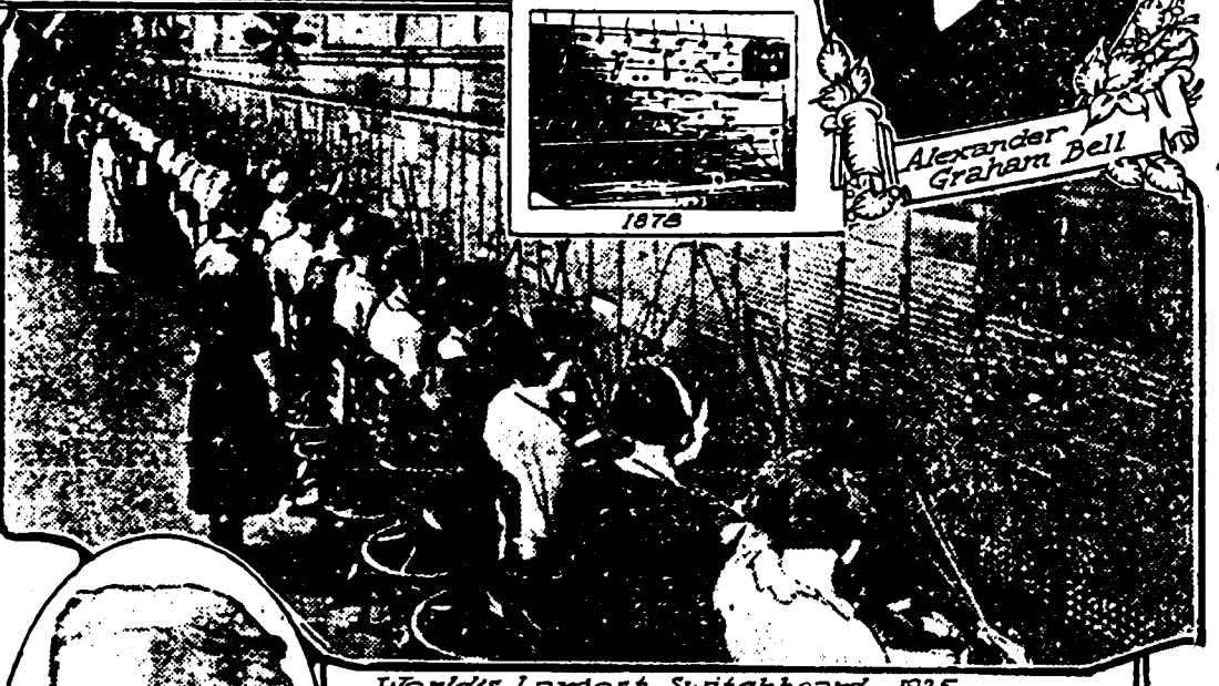
World's Largest Switchboard—1925
