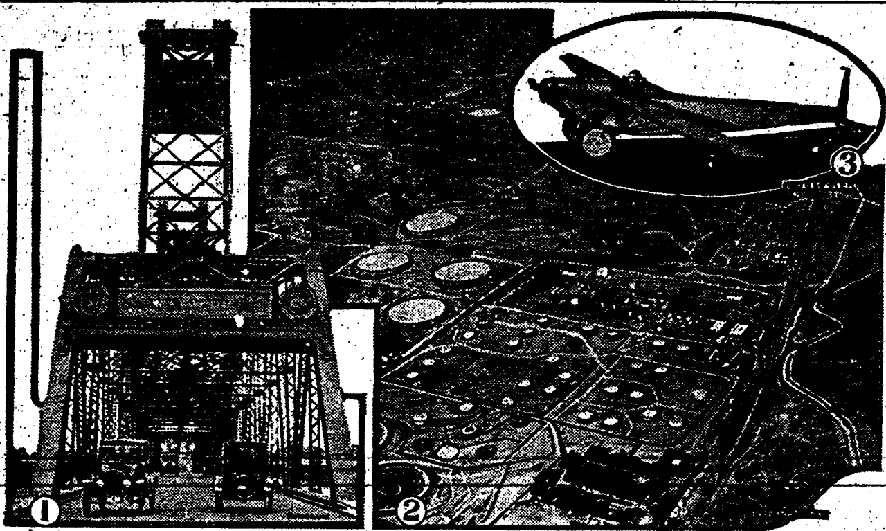
1—$2,000,000 bridge across the Piscataqua river, connecting Portsmouth, N. H., and Kittery, Me., erected as a memorial to the war dead of New Hampshire and Maine. 2—Airplane view of Elk Hills naval oil reserve in California, leases to which the government seeks to cancel. 3—E. F. Allen of Washington in his baby plane, weighing 205 pounds and capable of making 63 miles an hour.
