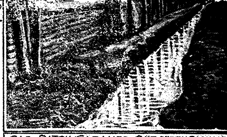
OLD DITCH CLEANED OUT WITH DYNAMITE
